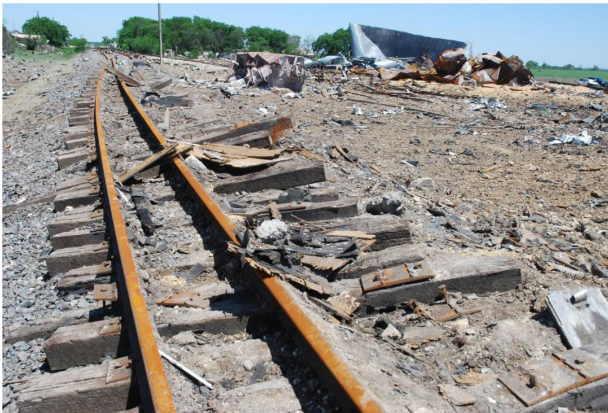
Railroad tracks displaced next to the blast seat.
